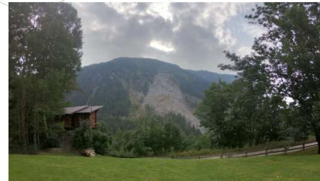
Complex, rockslides, deep-seated LS
